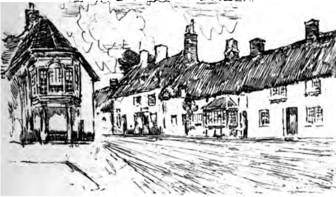
A Corner in Puddletown.
